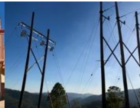
34.5kV powerline, 20km east
